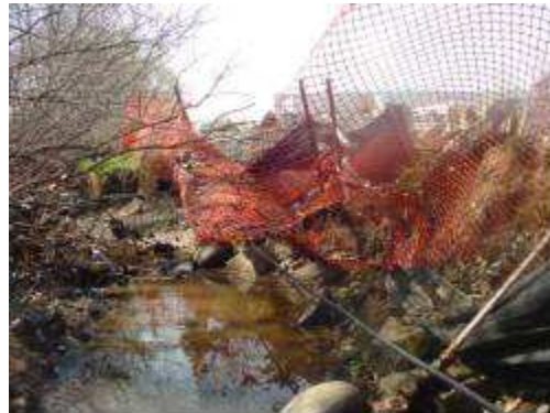
Figure 1.1 Damage on Pfizer Campus Along Millers Creek
